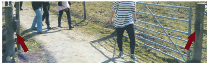
Protective Housing on gate posts
